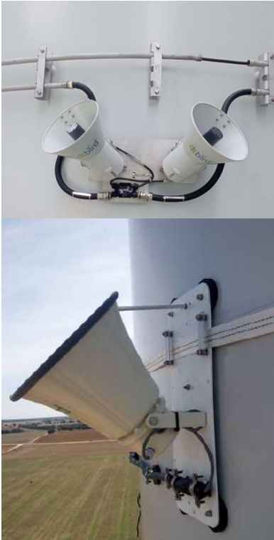
DTBird Collision Avoidance Module Speakers installed on the WTG tower. 4 to 10 Speakers can be installed per WTG.
