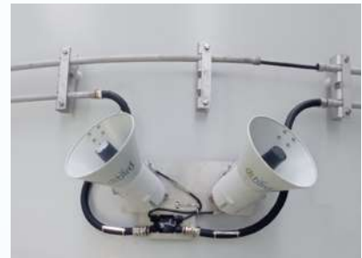
DTBird® Collision Avoidance Module Speakers installed on the WTG tower. 4 to 10 Speakers can be installed per WTG.
