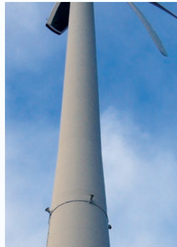
DTBird® Collision Avoidance Module installed in France. View of 3 of the 4 Speakers.
